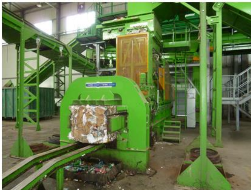
Figure A1-2: Front End of Waste Sorting Line
