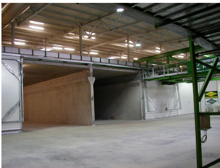
Figure A3-3: In-Vessel Composting (IVC) System
