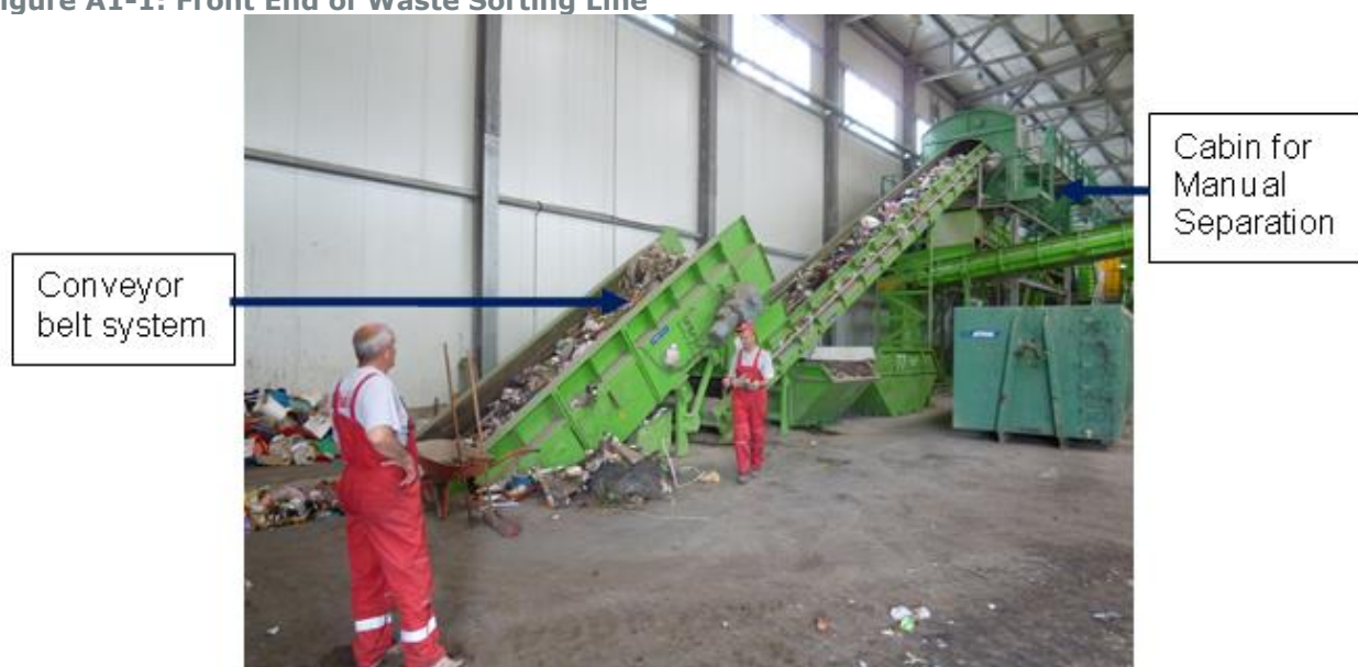
Figure A1-1: Front End of Waste Sorting Line
